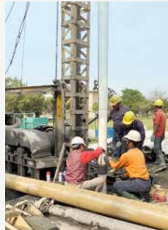
鑿井工程 Well drilling engineering
